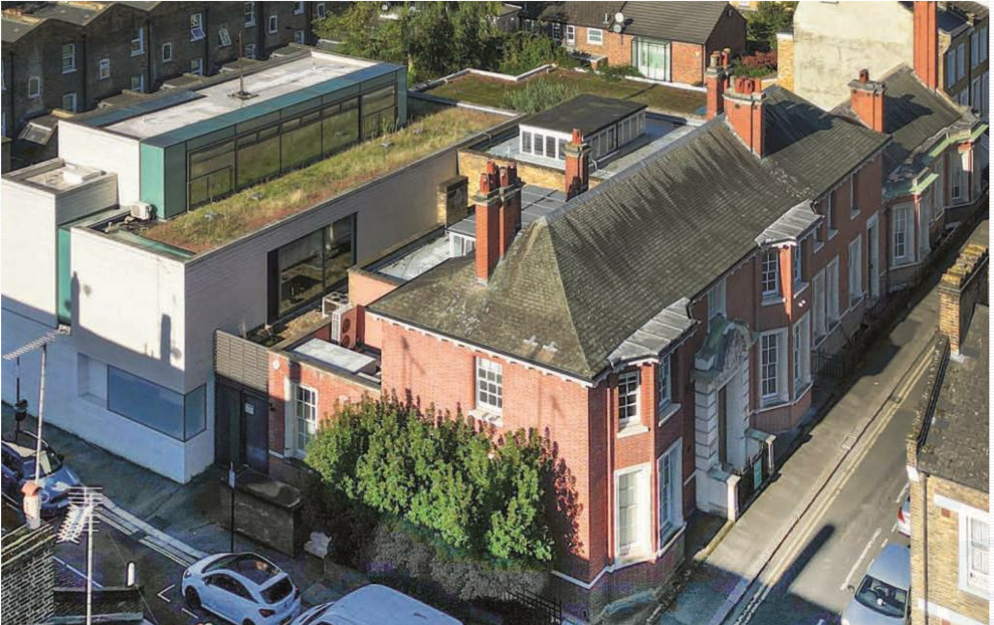
Vernon Street & 10 Southcombe Street, West Kensington, W14 0RA
