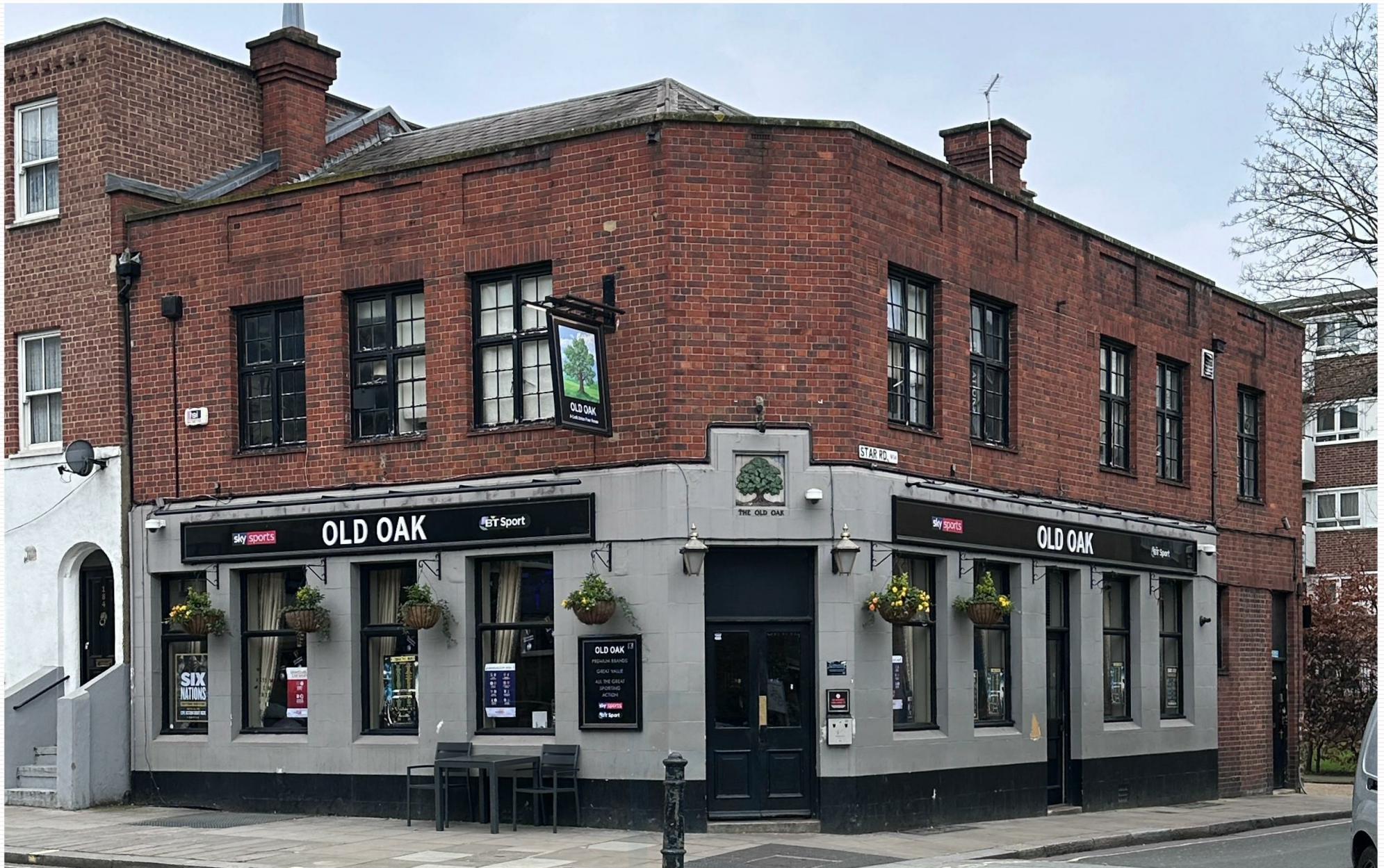
North End Road, West Kensington, W14 9NX
