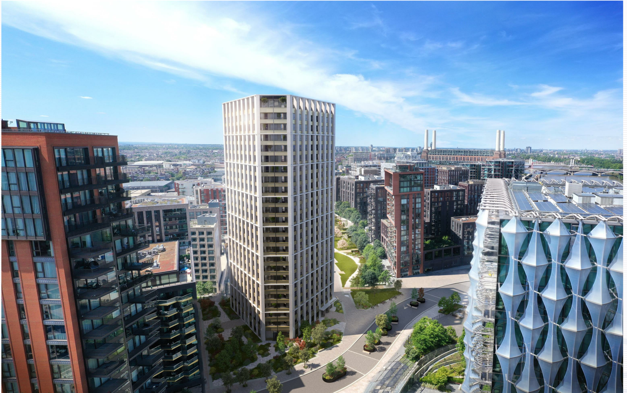
Penthouse Apartments, Ascenta, Nine Elms, SW11
