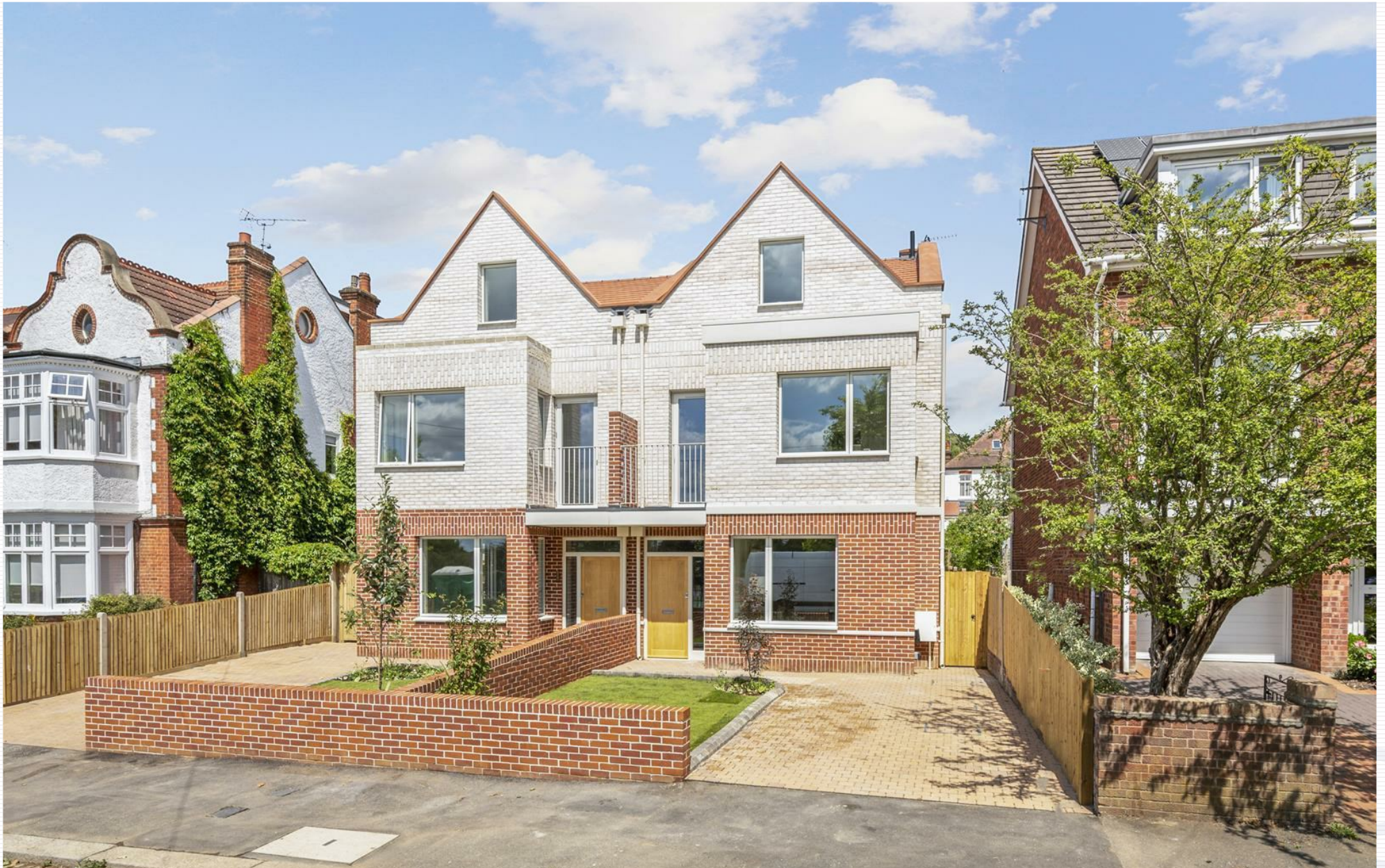
Melbury Gardens, West Wimbledon, SW20 0DJ
